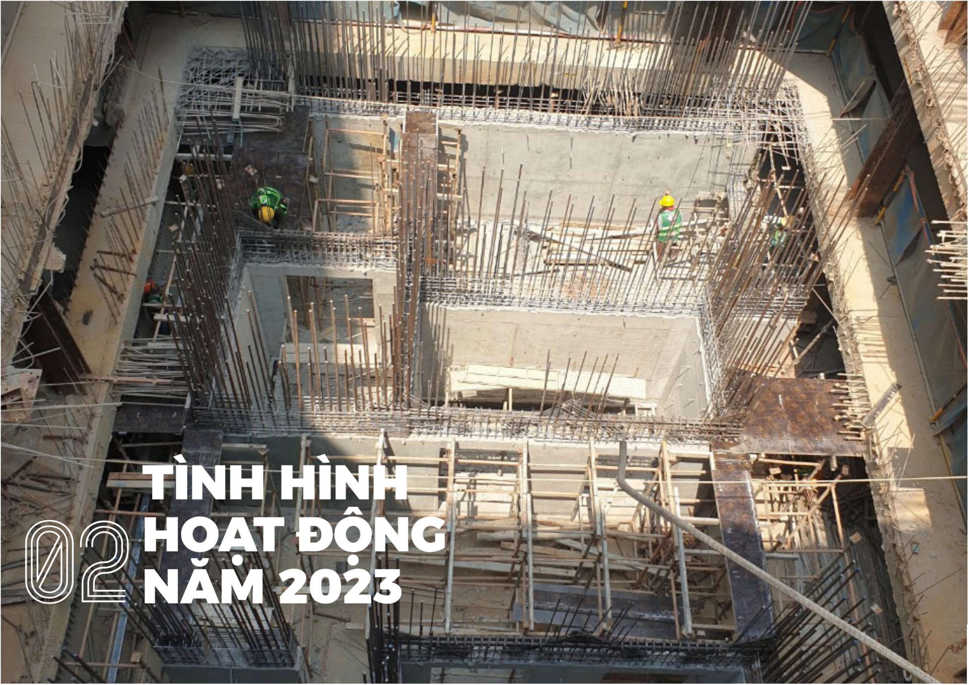
The background image shows a massive construction site, likely for a skyscraper, with extensive steel reinforcement bars (rebar) and wooden formwork. Several workers wearing hard hats and safety vests are visible on the scaffolding and working on the concrete structures.
